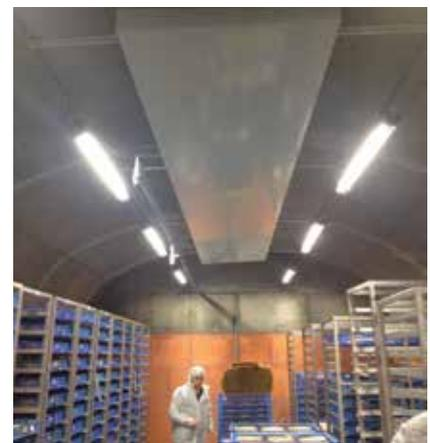
*A static cooling system that circulates cold water around radiator fins to cool the air. The cool air then falls under gravity. A vaulted ceiling assists in the airflow.*
